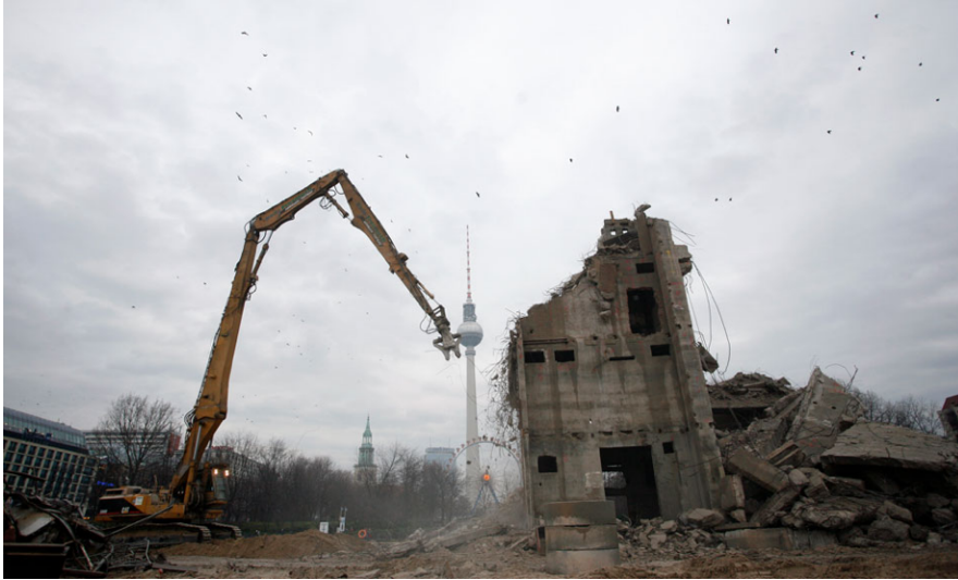
Demolition crews finish off the Palace of the Republic in Berlin in December 2008. After unification, the new German government sought to erase all reminders of the socialist GDR. The apartments along Karl Marx Allee, however, proved to be too well-constructed to be demolished so easily. | Miguel Villagran / AP
